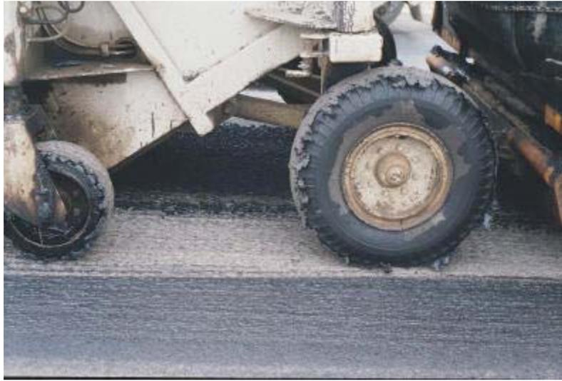
Tack coat tracking resulting in no tack coat in the wheel path.
